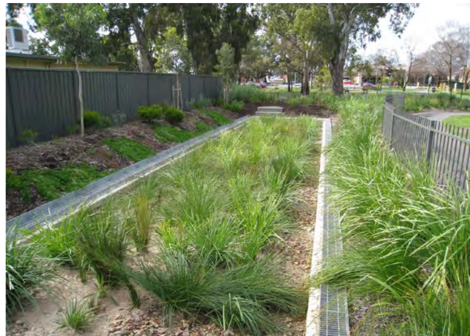
BIO-FILTRATION CELL AT LINDE RESERVE
