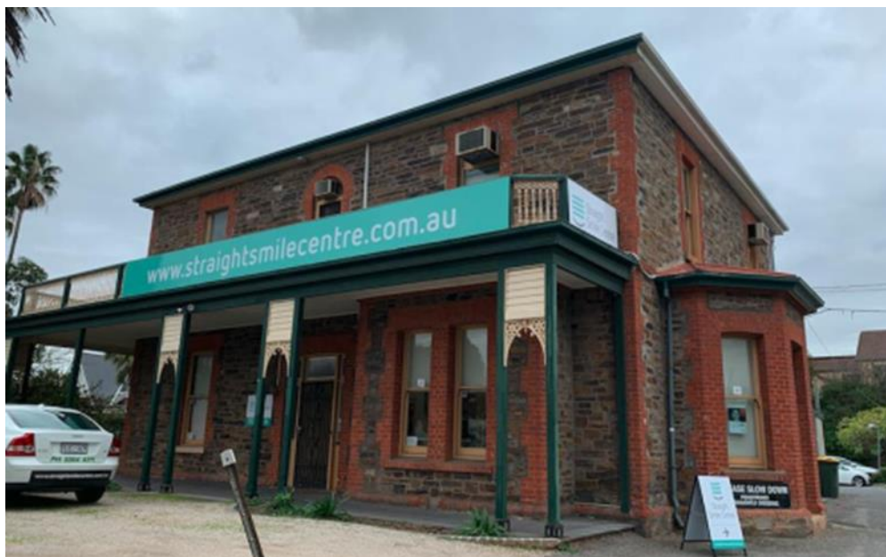
Figure 5.3 - 139 Kensington Road, Norwood: Victoria Bluestone Two-Storey Building
