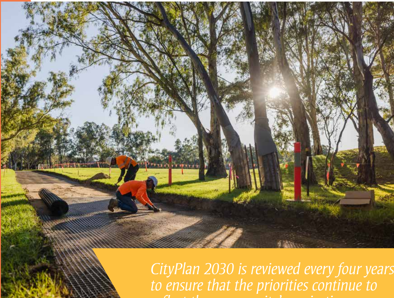
River Torrens Linear Park Shared Path
