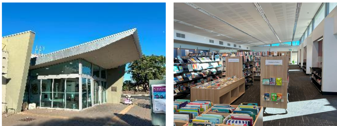
Figure Five: Payneham Library – contemporary entranceway and congested floor area with high shelving
