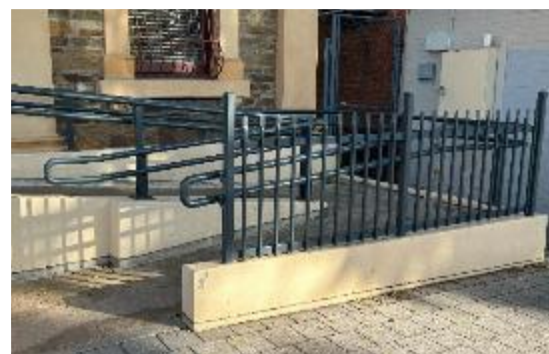
Figure Four: Norwood Library – front access ramp
