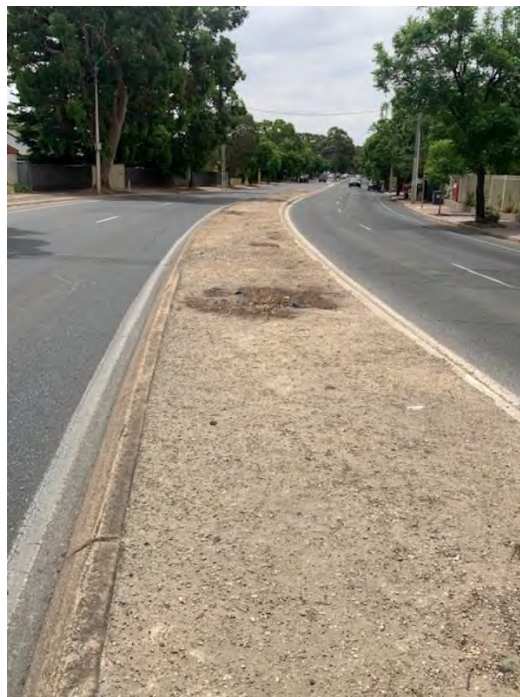
OG Road (between Turner St and Pitt St looking north)
