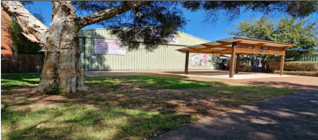
17. St Peters Rotary Shed 46A Henry Street, Stepney
