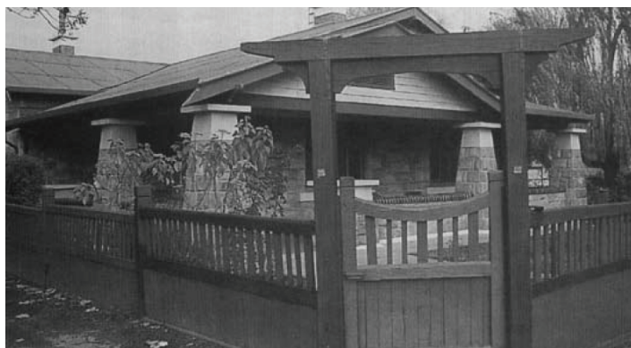
A typical timber picket Bungalow fence.
