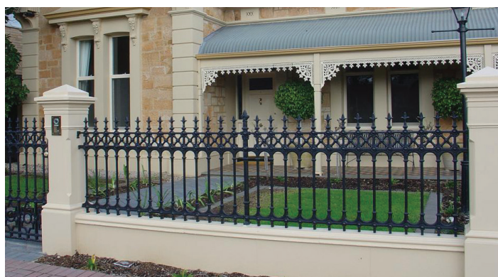
A St Peters masonry front fence with cast metal infill.
